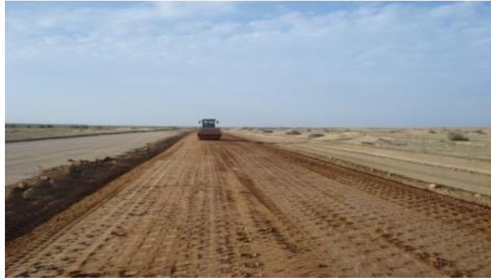
Figure (8) - Operation of pounding embankment layers for implementation
