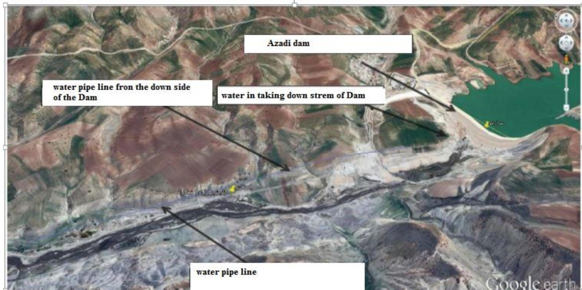
Image (3) of the route profile of the water transmission line from Soy to Har Plain
