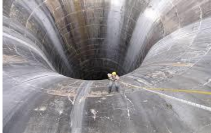
Image (3) the view of huge dimension of morning glory spillway
