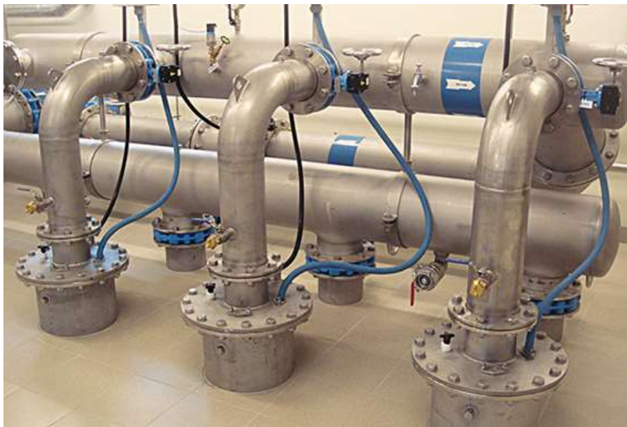
Figure 3. Vertical pumping station using floating pumps.
